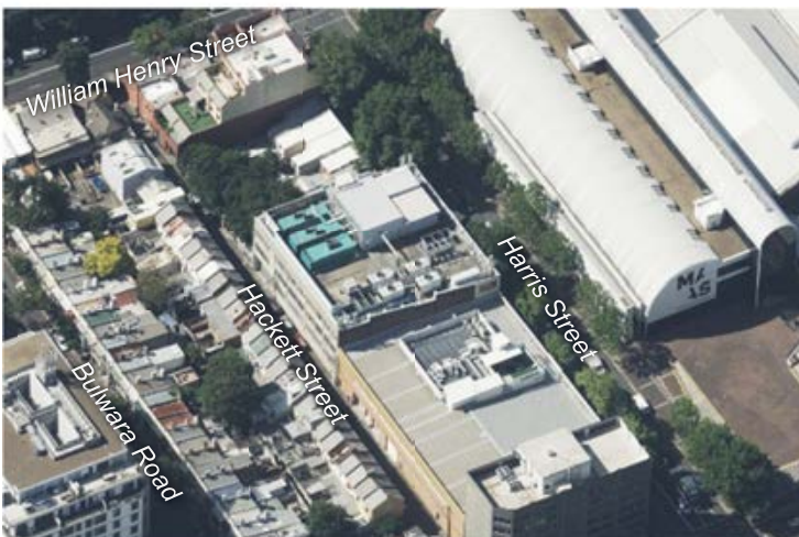
Figure 164 – oblique aerial of 549-559 Harris Street
