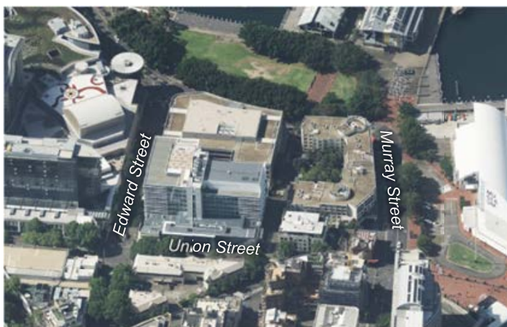
Figure 21 – oblique aerial of 2 Edward Street & 60 Union Street
