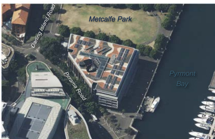
Figure 113 – oblique aerial of 48 Pirrama Road
