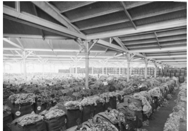
Top floor interior of 28-48 Wattle Street (Winchcombe Carson Ltd) c. 1901 Source: Museums of History NSW, NRS-4481-3-[7/16281]-St1527
