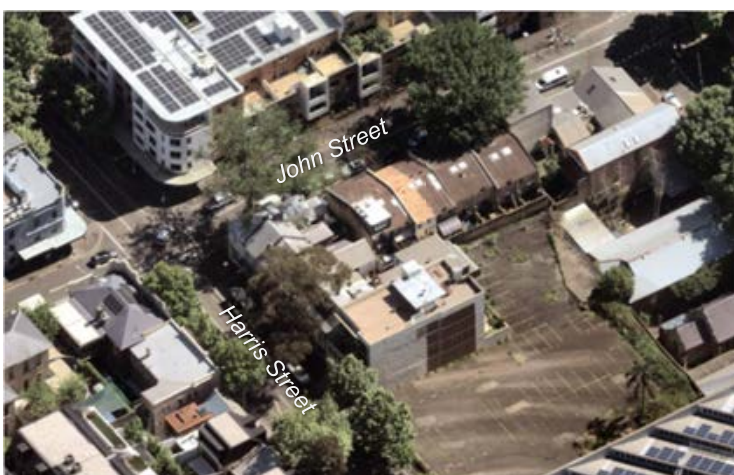
Figure 91 – oblique aerial of 80-84 Harris Street
