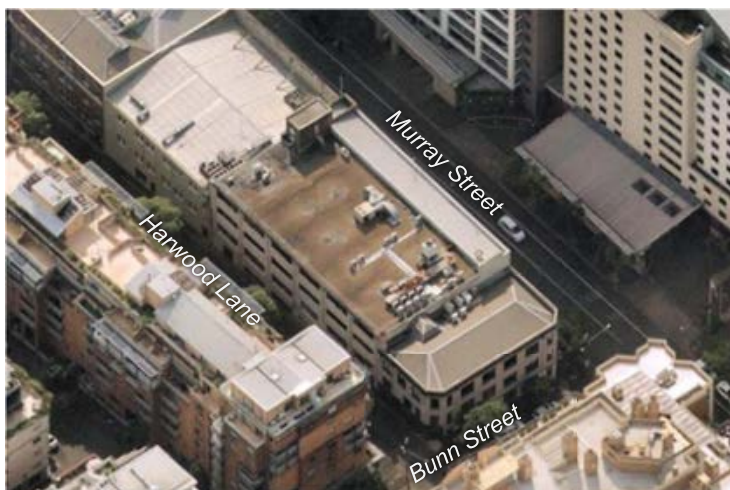
Figure 56 – oblique aerial of 55-65 Murray Street
