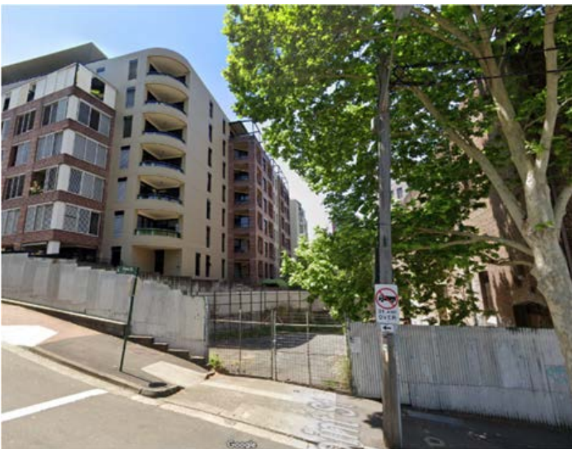
Figure 106 – Watermark Apartments, overlooking the view corridor (source: Google StreetView)
