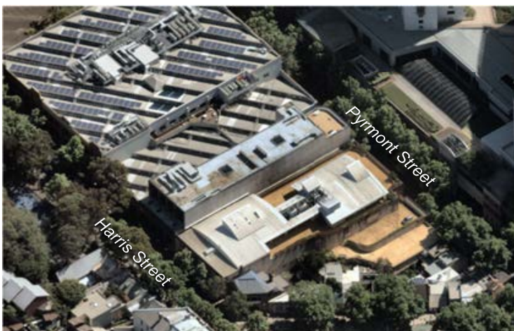
Figure 122 – oblique aerial of 100 Harris Street
