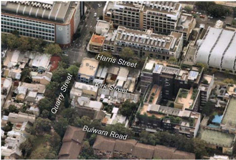
Figure 152 – oblique aerial of 469-483 Harris Street
