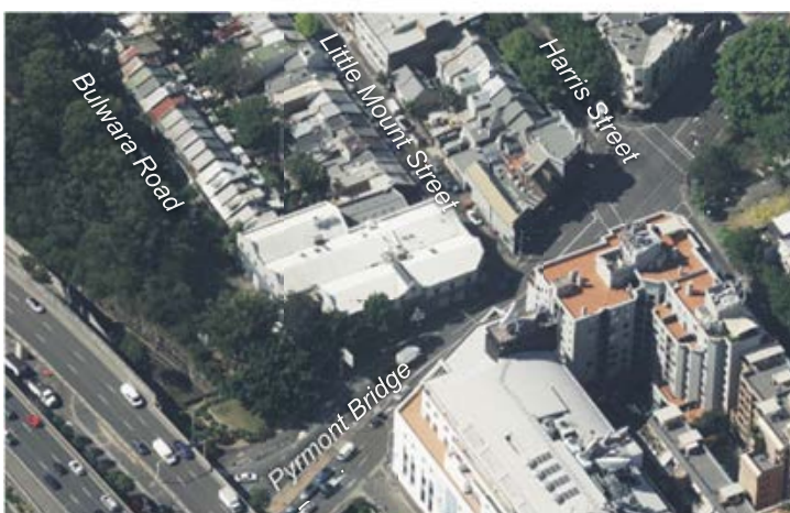
Figure 2 – oblique aerial of 46-48 Pymont Bridge Road
