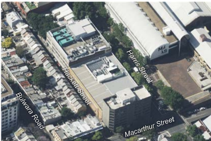
Figure 170 – oblique aerial of 561-577 & 579-583 Harris Street
