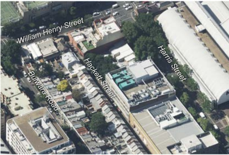
Figure 158 – oblique aerial of 535-547 Harris Street
